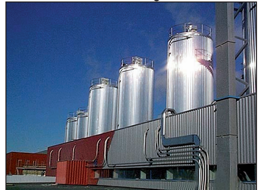
Silos / Coating silos
